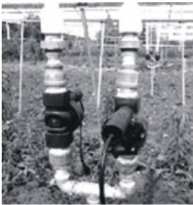
Install the valve in the pipe net. Make sure water in the valve will not freeze, that the water is clean, and pressure changes when the valve opens or closes will not cause water hammer..
