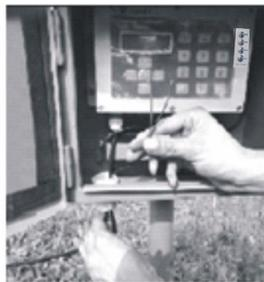
Put the valve connection wire into the box, choose correct terminal on the controller and remove it.
